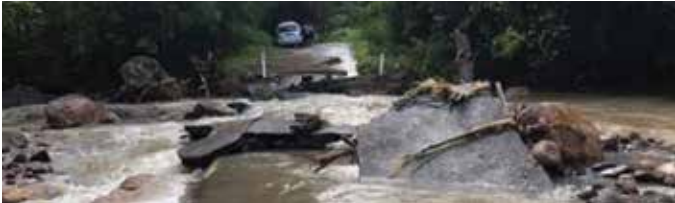
Pictured: Section of Wilsons Creek Road, post flooding.
