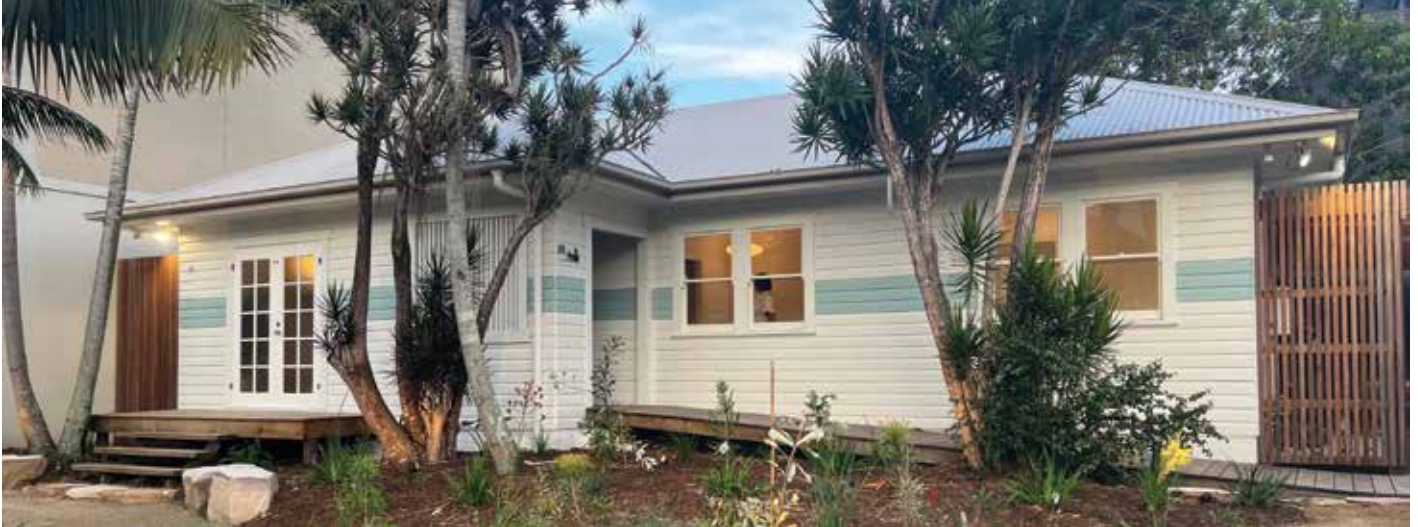
Pictured: Fletcher Street Cottage post renovation. Source: Byron Community Centre
