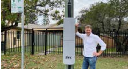
Pictured: Mayor Michael Lyon at EVX pole charger on Wordsworth Street. Source: EVX.
